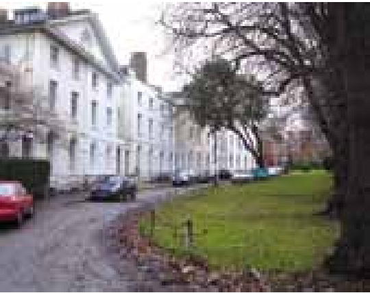
169 to 183 Grove Crescent
