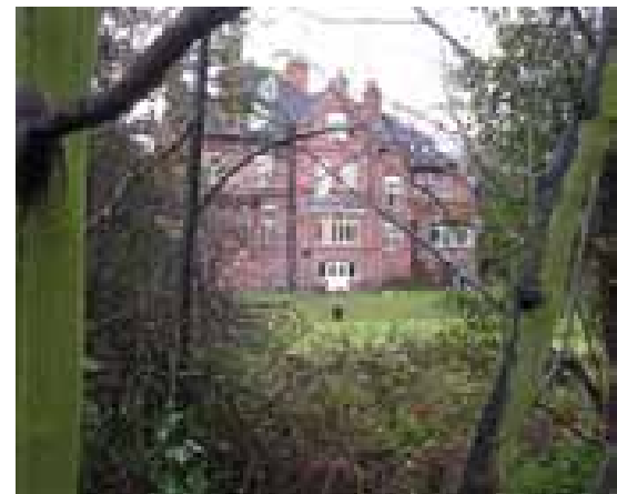
123 Grove Park from the south
